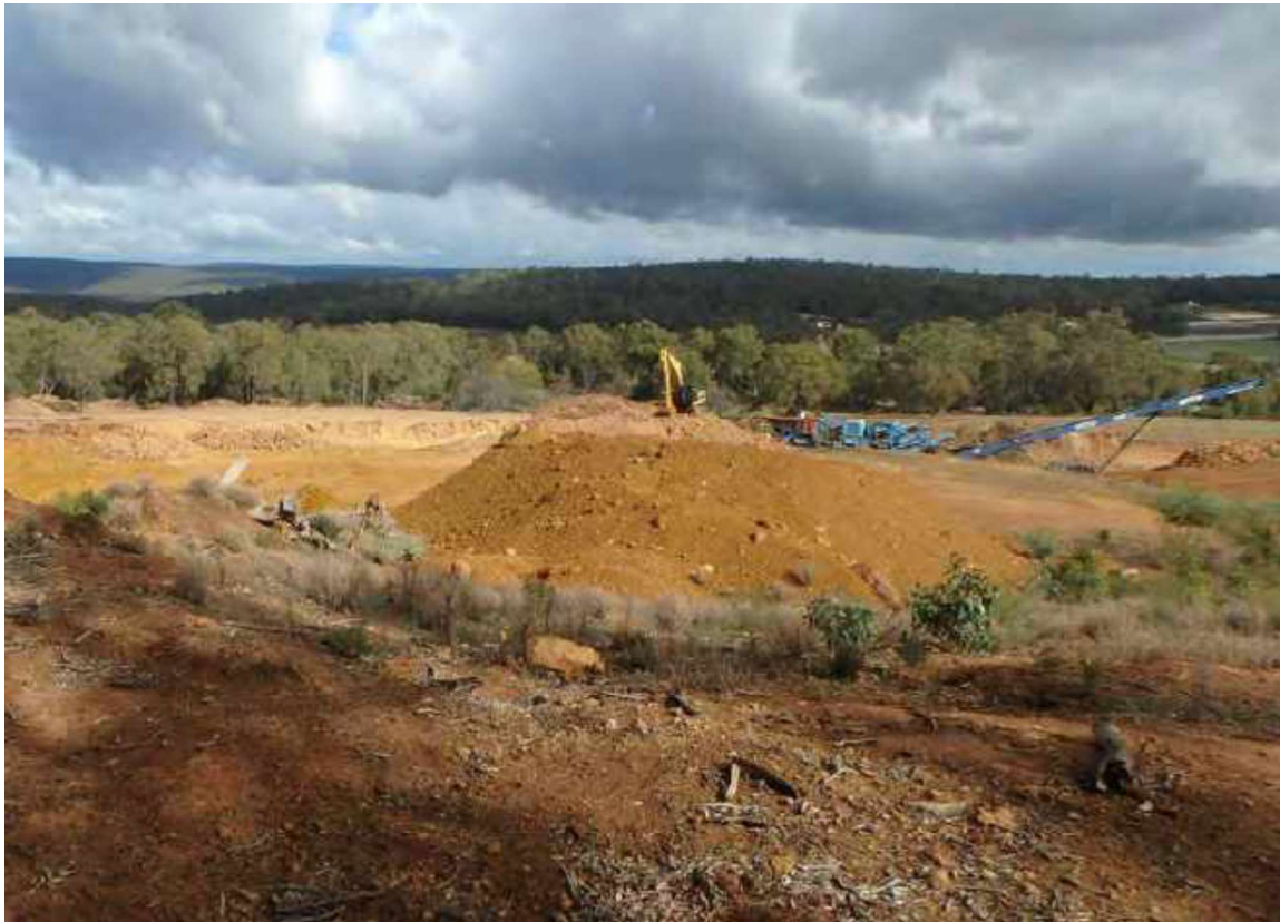
Plate 7: Cleared in 'completely degraded' condition
